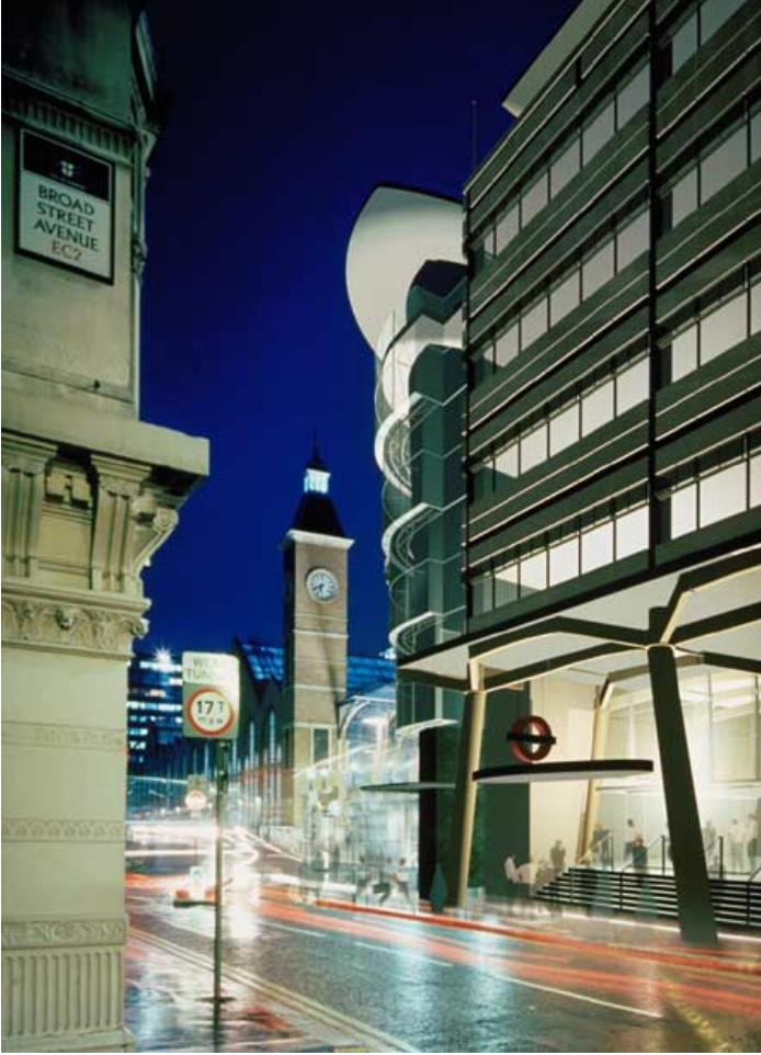
Exhibit 17 Liverpool Street Station, London
