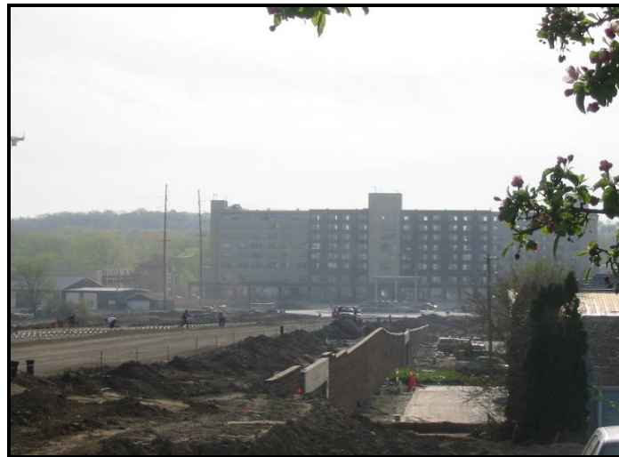
Convention Center under construction in Coralville.
