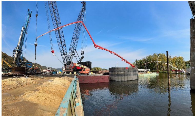
Concrete Pumps for Drilled Shafts
