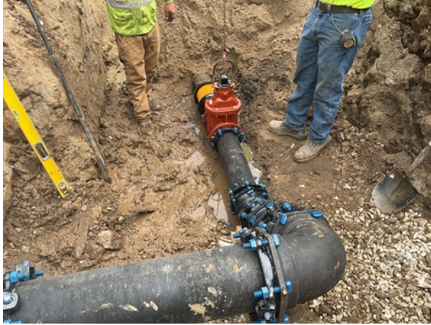
Water Line Replacement
