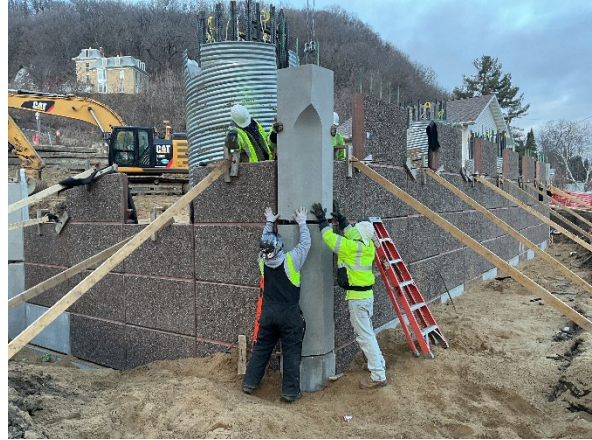
MSE wall in Lansing
