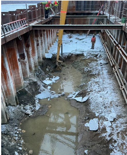
Pier 1 cofferdam clean up
