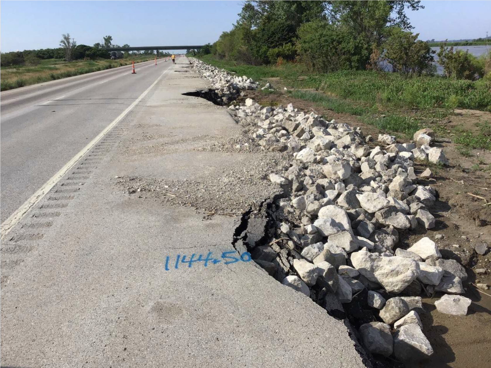
“Rip rap protects the remaining facility”
