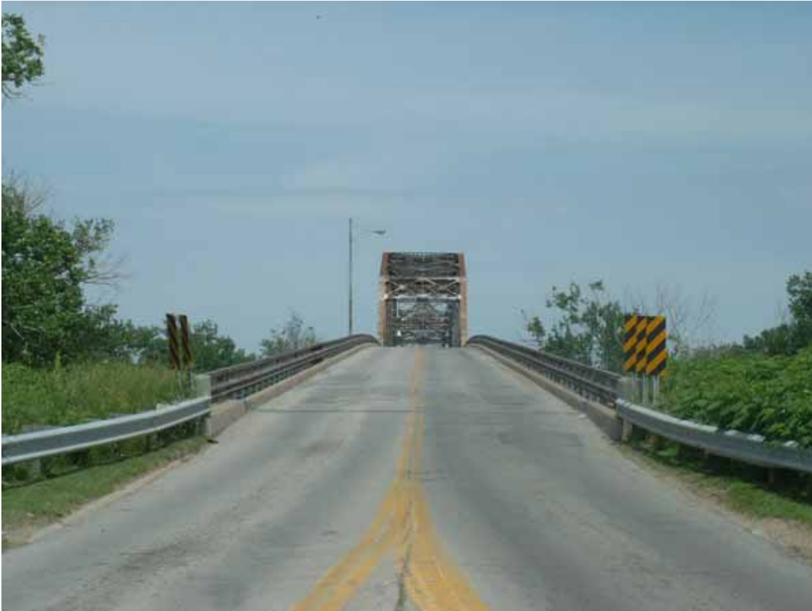
Figure 1-3 Existing Bellevue Bridge
