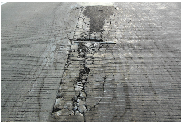
Concrete slab spalling.
