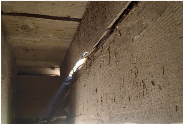
Cracked timber stringers.
