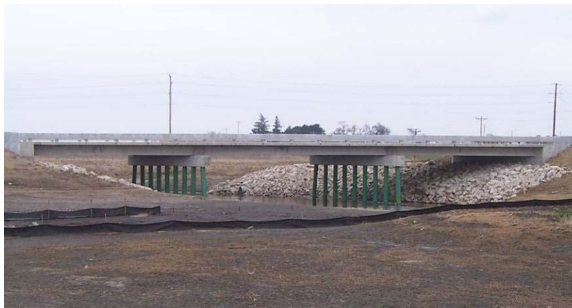
Figure 1.2 Completed replacement bridge on 120th St
