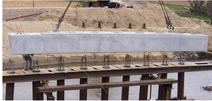
Figure 116. West pier cap being lowered into place, October 4
