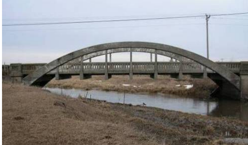
a) Replaced Marsh Arch bridge
