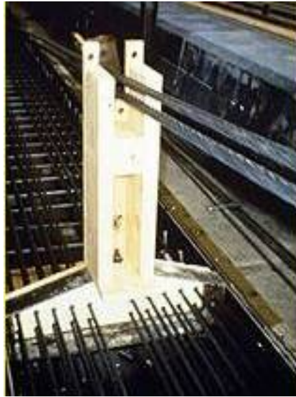
Figure 3. Bulkhead in a prestressed concrete casting bed
