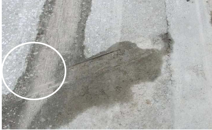
Figure 148. Low area in one transverse joint after deck grinding, December 27
