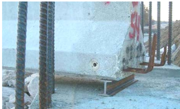
Figure 125. Steel beams used to support the girders, October 24
