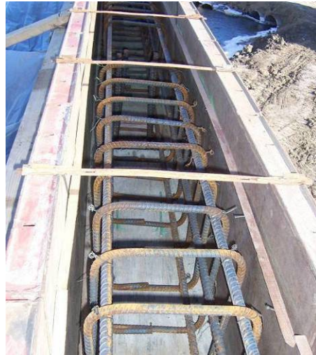
Figure 144. Barrier rail reinforcement, December 8
