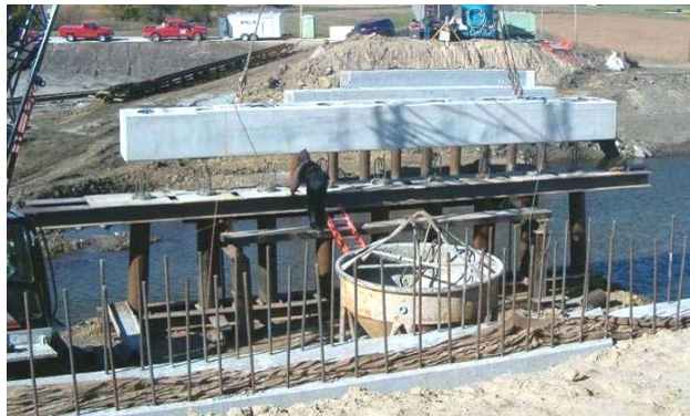
Figure 123. East pier cap being set, October 12
