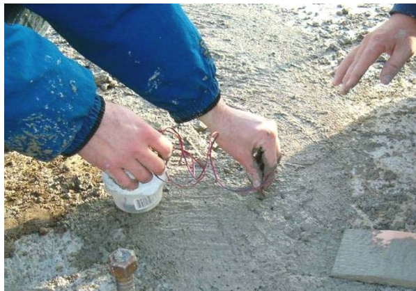
Figure 135. Thermal couple being inserted into end panel joint, November 16
