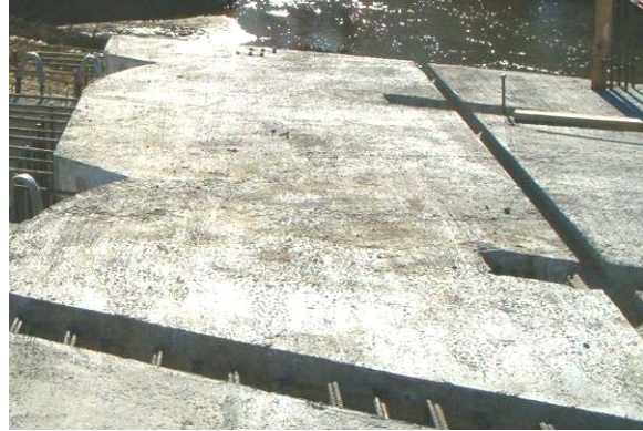
b) complete end panel in the field
