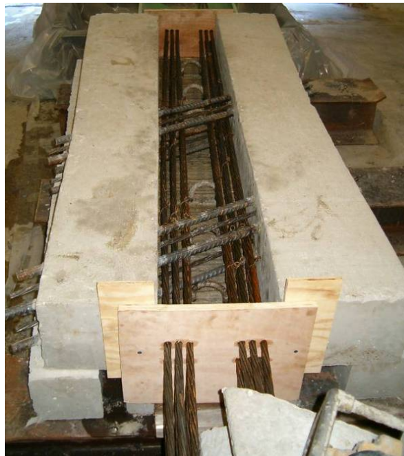
a) Constructed channel used in concrete placement tests (courtesy of Iowa DOT)
