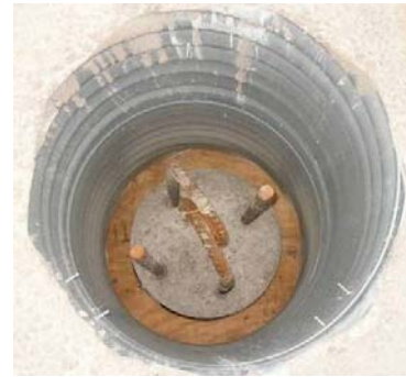
b) pipe pile in the pier cap
