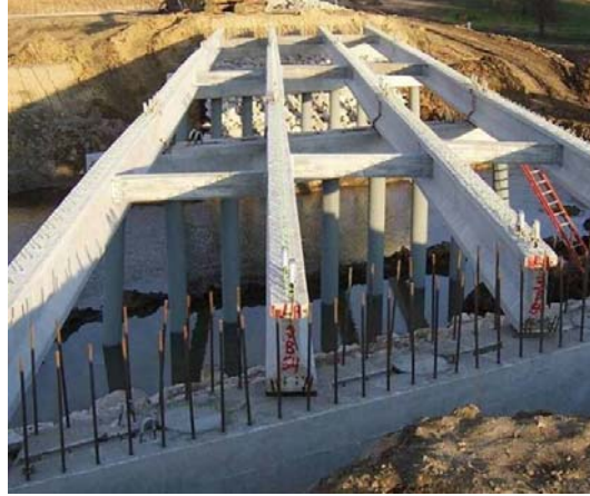
Figure 126. Erected bridge girders, October 24
