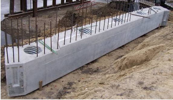
a) abutment in final position
