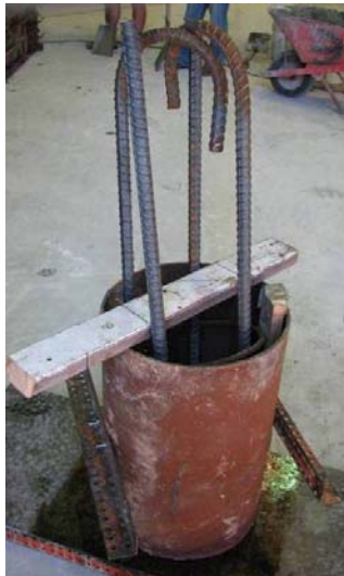
a) Pipe pile before placing concrete
