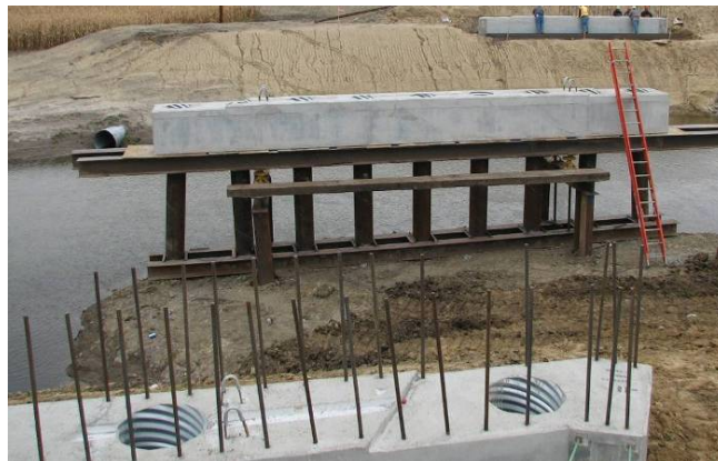
Figure 118. Precast abutments and pier cap in place, October 4
