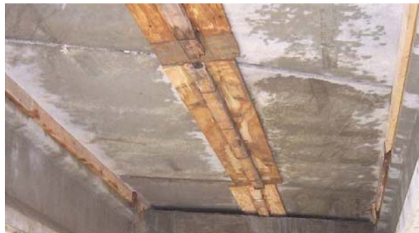
Figure 139. Longitudinal joint formwork, November 28
