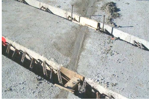
Figure 134. Finished transverse joint, November 8
