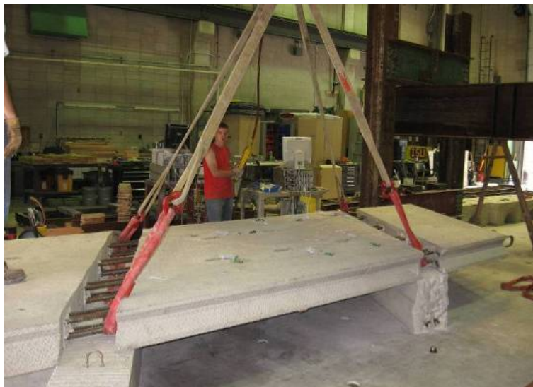
a) Photograph of two strap setup prior to lifting
