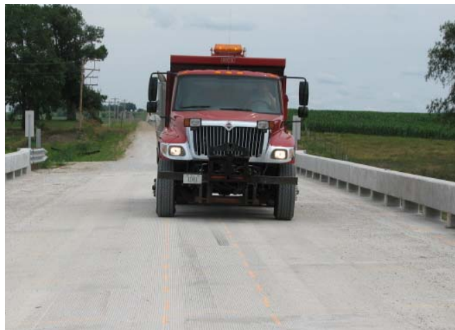
Figure 2.10 Test vehicle in Lane 3 position
