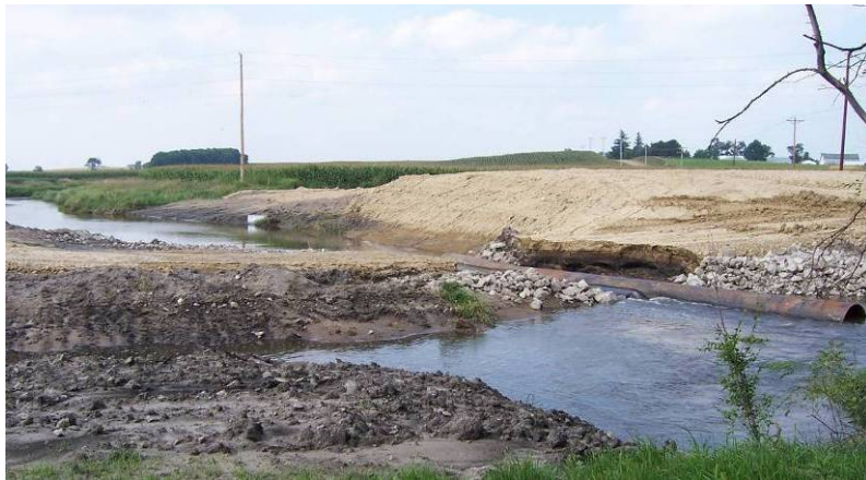
Figure 104. Access road and bridge site, August 11
