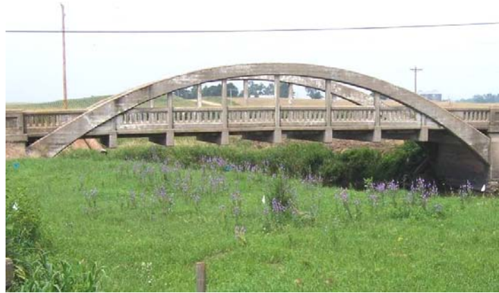
Figure 1. Marsh Arch bridge previously on 120 th Street
