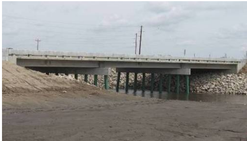
b) Completed replacement bridge
