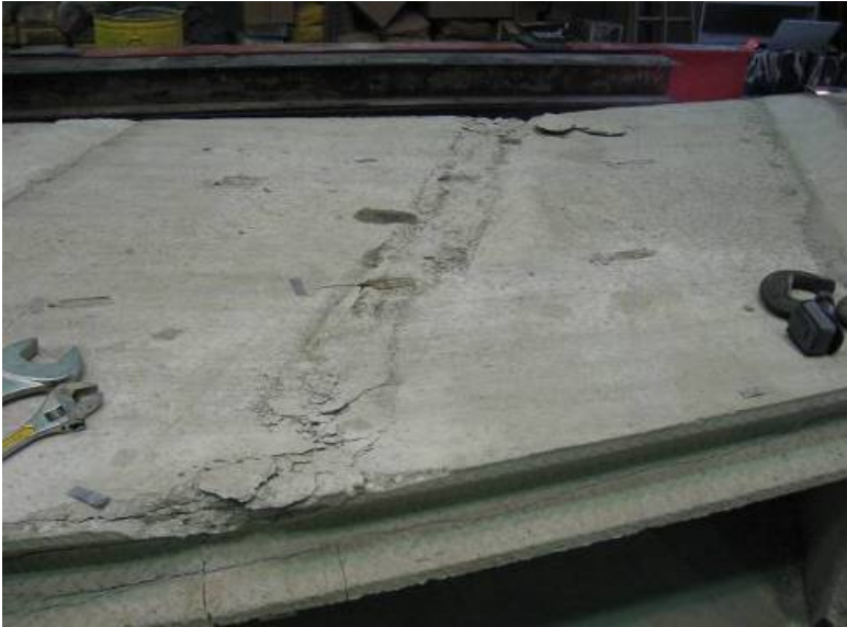
a) Deck panel after loading
