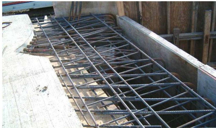
Figure 141. Reinforcement in the west abutment cap, November 29
