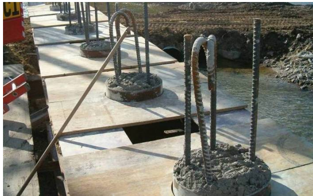
Figure 122. East pier pipe piles filled with concrete, October 12
