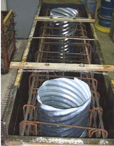
Figure 32. Finished reinforcement and formwork for ADC1
