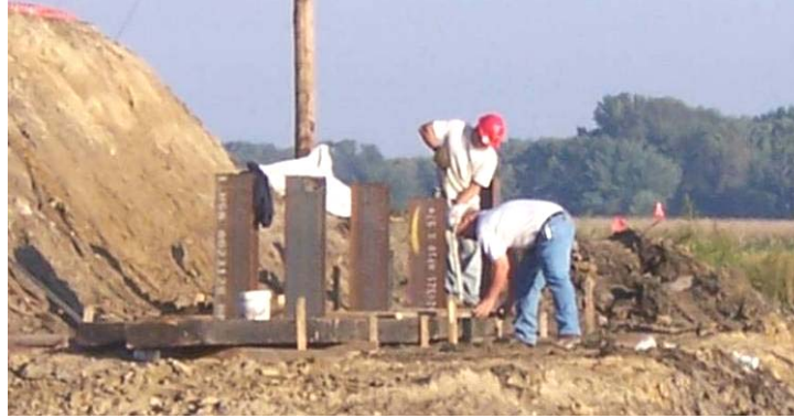
Figure 107. West abutment piles, driven and channels being blocked, September 15
