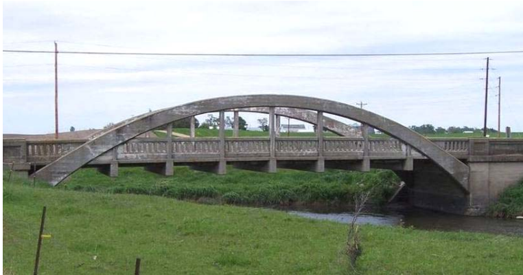
Figure 100. Previous bridge on 120 th Street, July 19
