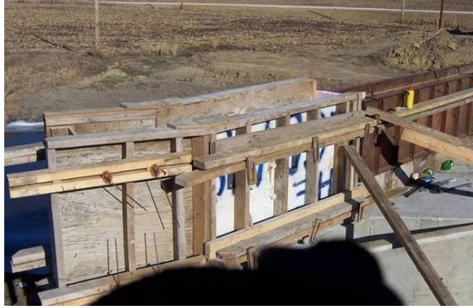
Figure 143. Barrier rail formwork, December 8
