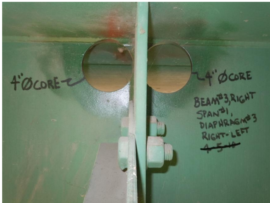
Figure 6.2.10-1. Diaphragm Connection Stiffener Fatigue Crack Retrofit
