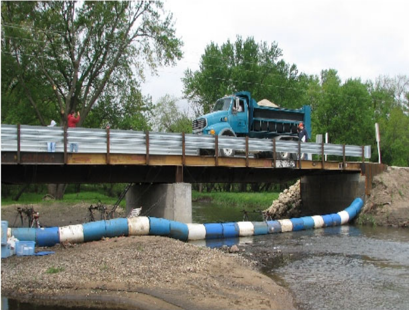
Figure 2. BCB5 RRFC Bridge Test (May 11, 2006)
