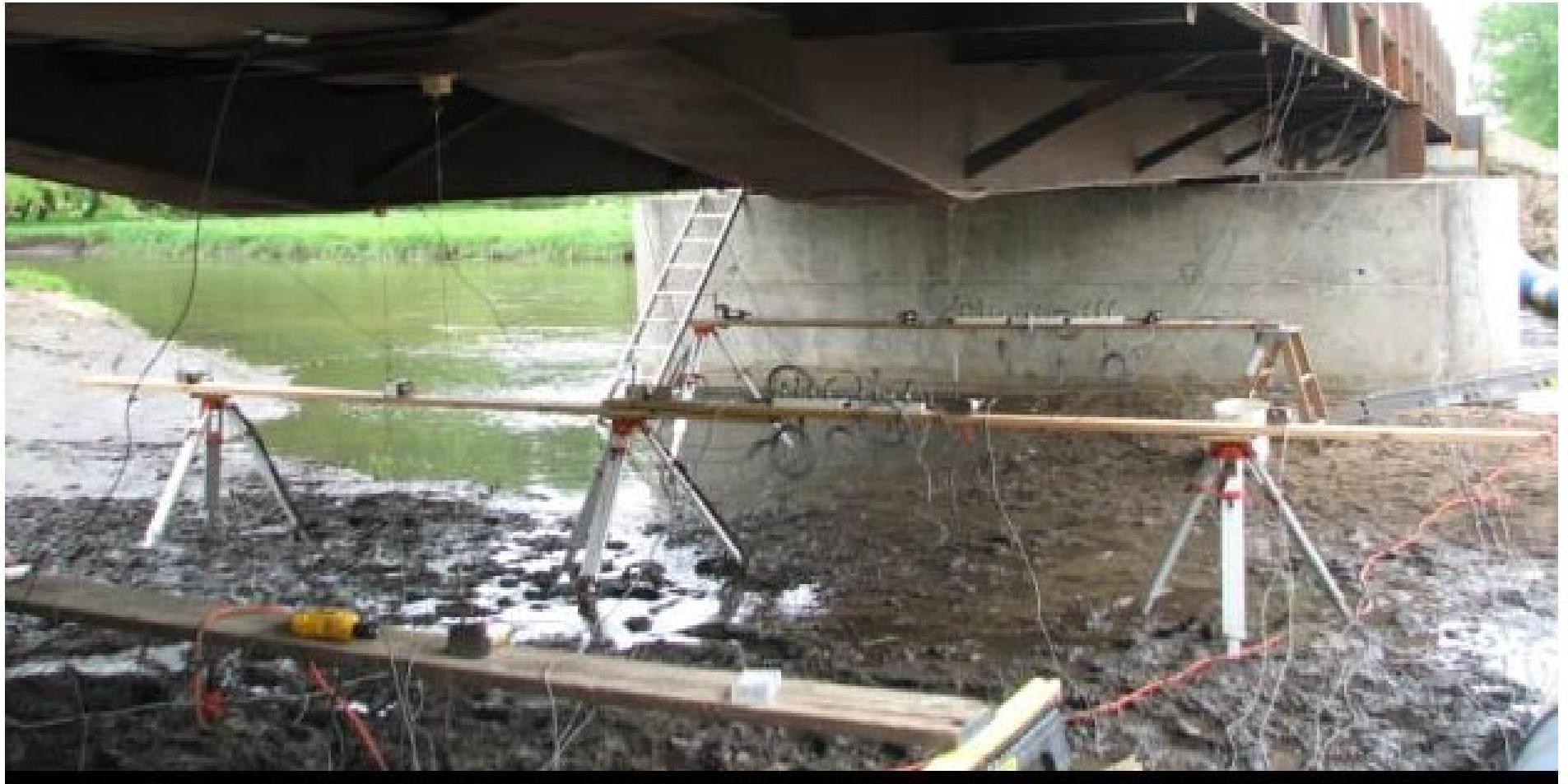
Figure 1. BCB5 RRFC Bridge Test Instrumentation (May 11, 2006)
