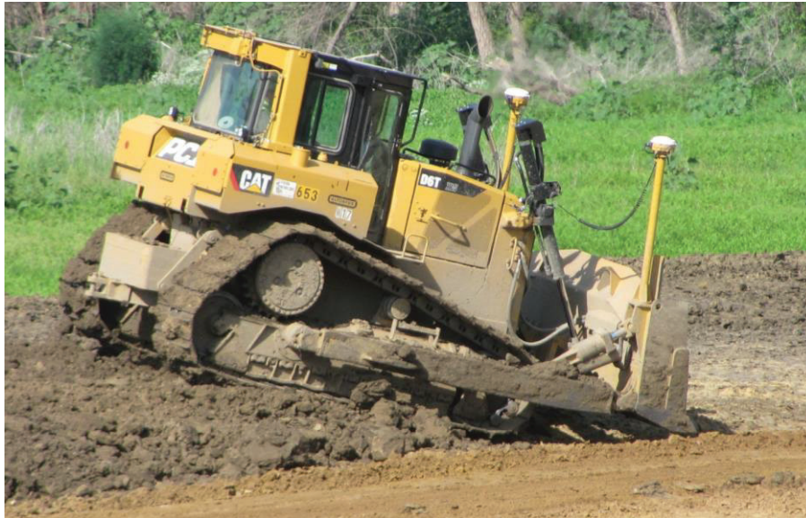
Figure 6-2: The Contractor must construct embankments uniformly and in lifts not to exceed 8-inches in loose thickness.
