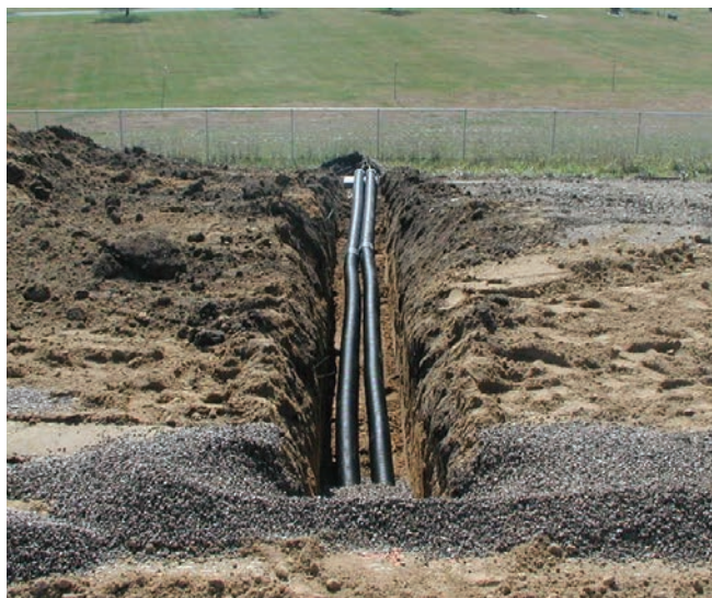
Figure 9-6: Longitudinal subdrain outlets
