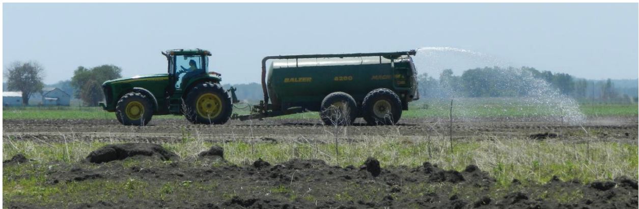
Figure 4-5: Water truck applying water to reduce dust
