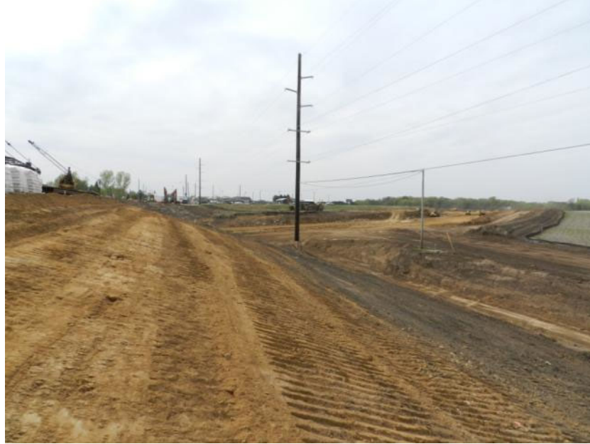
Figure 5-1: Grading may occur around existing utilities.
