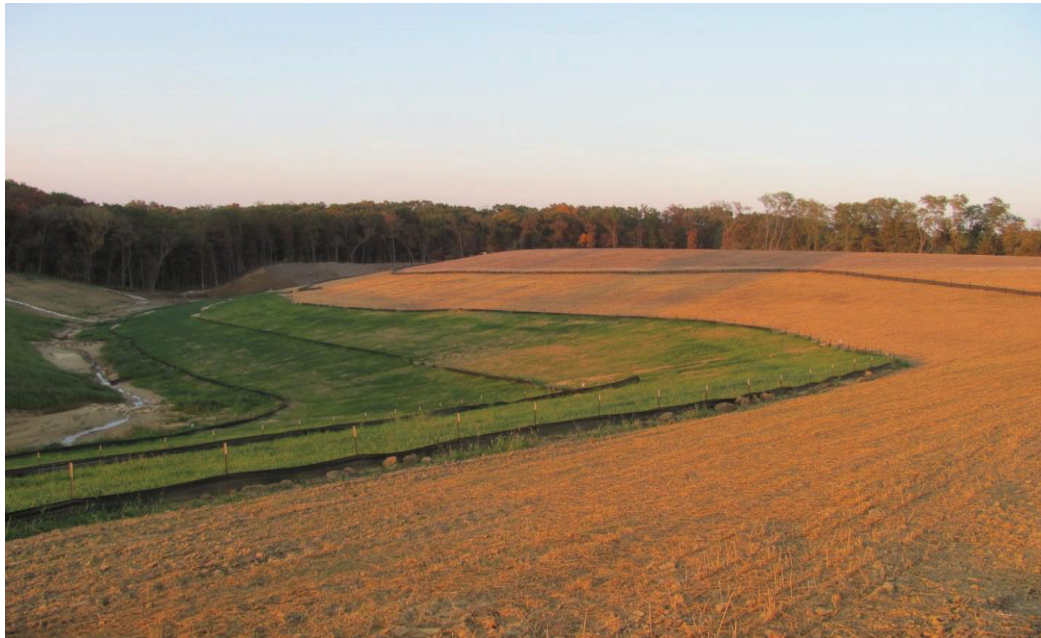
Figure 11-3: Staged seeding is a good practice to reduce erosion.
