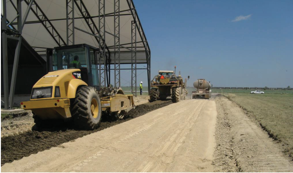
Figure 10-3: Compaction following behind pulverizer.
