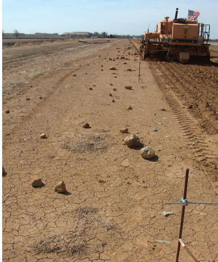
Figure 6-4: Rocks that required removal prior to paving
