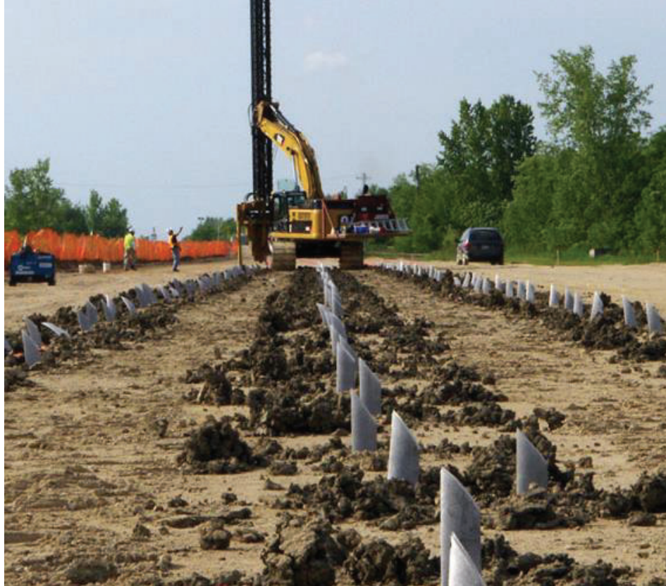
Figure 9-8: Rows of installed wick drains
