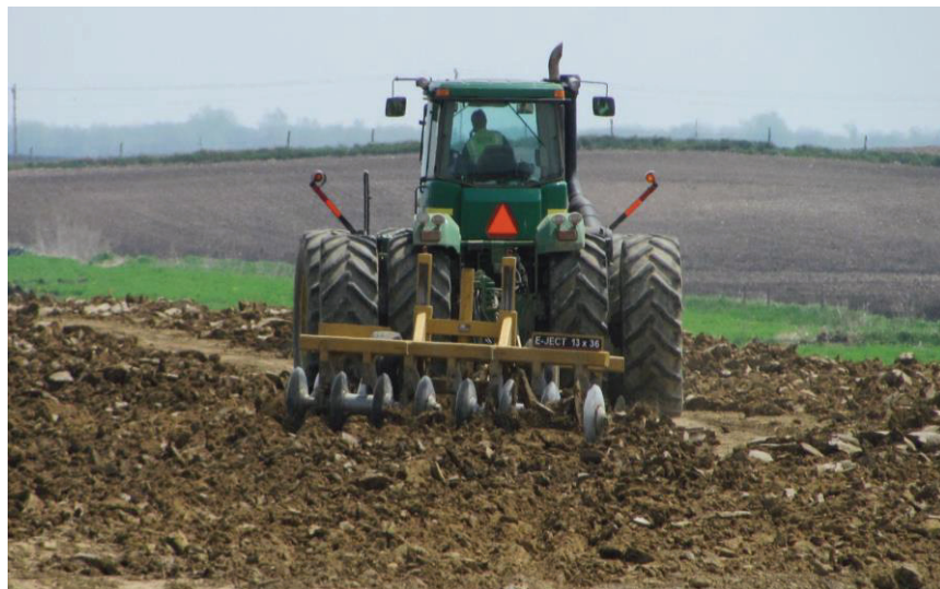
Figure 6-5: Disking helps break up clods that would prevent uniform compaction.
