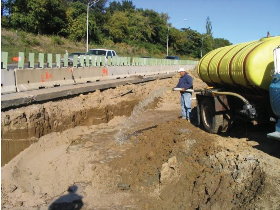
Figure 8-5: Applying water to flooded backfill
