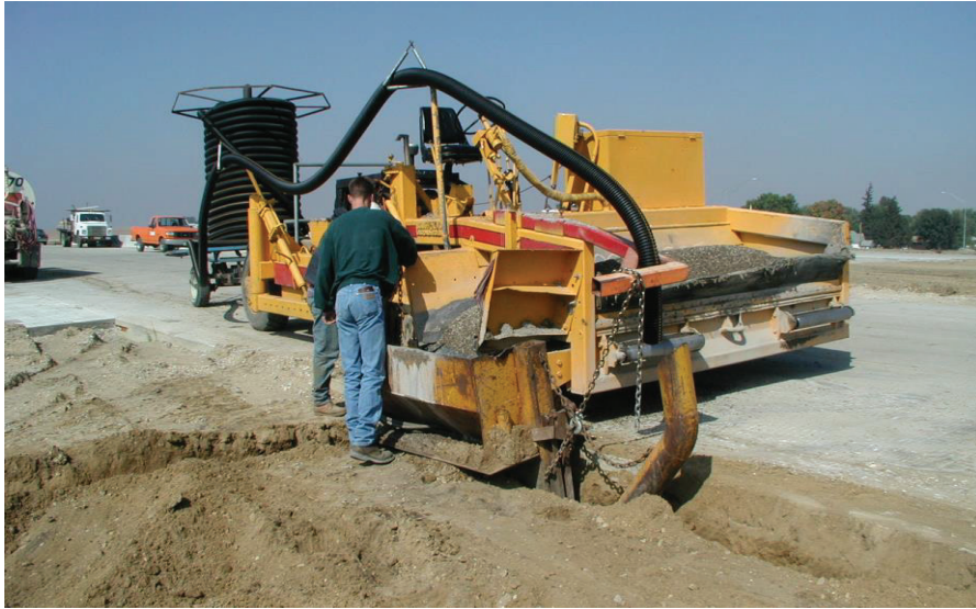
Figure 9-5: Installation of longitudinal subdrain
