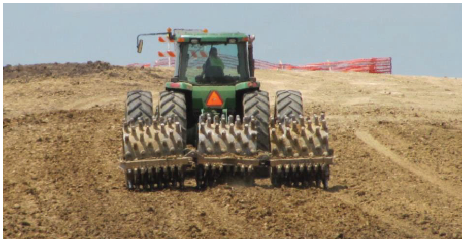
Figure 4-8: Sheepsfoot roller pulled by tractor
