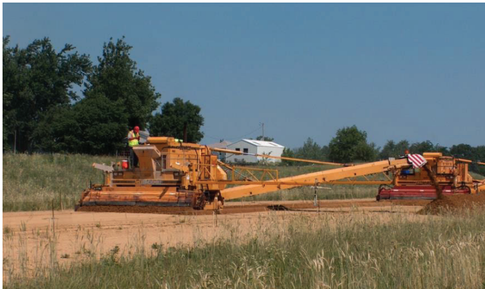
Figure 12-3: Subgrade trimming operations
