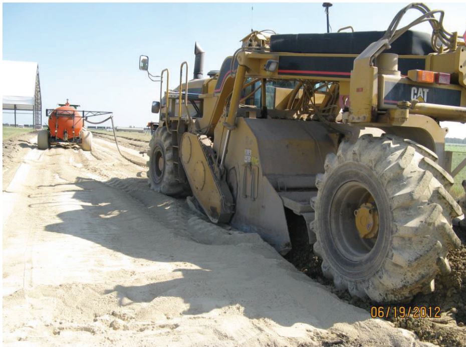
Figure 10-2: Pulverizer mixing fly-ash with subgrade soil.
