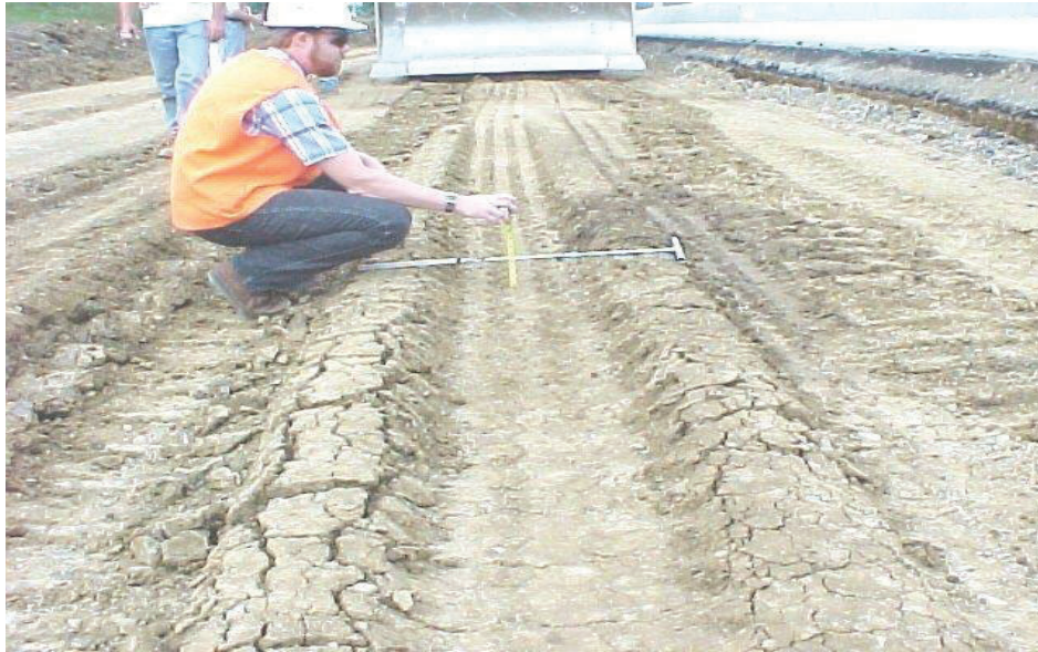
Figure 12-1: Inspector measuring ruts following the proof-roll test.
