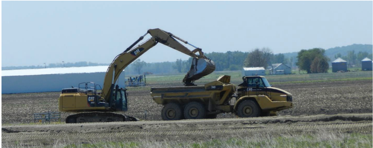
Figure 4-4: Excavator (backhoe) loading a truck
