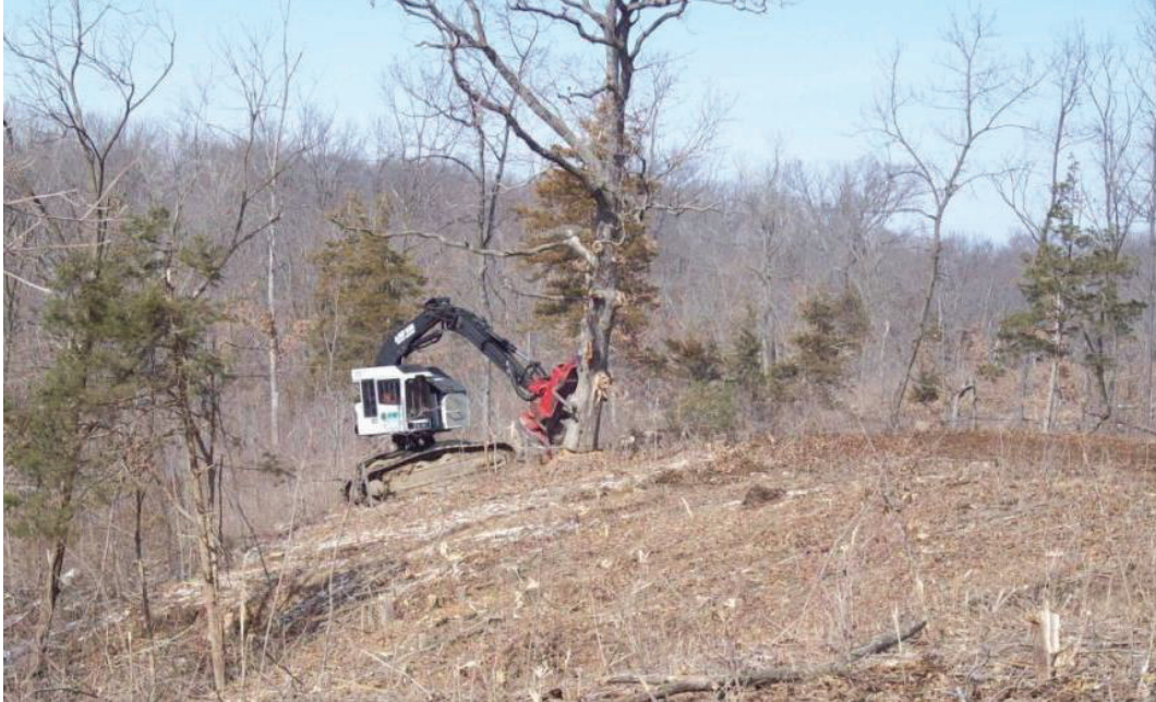
Figure 5-1: Clearing of trees
