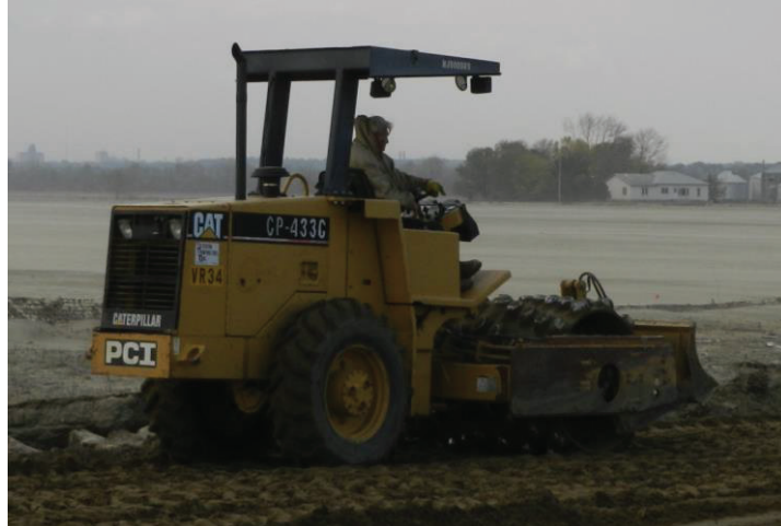
Figure 4-9: Pad-foot vibratory roller compacting granular soils.
