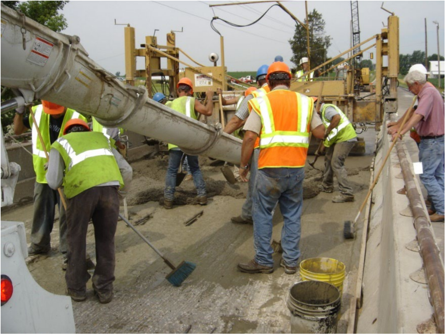
Bridge Deck Overlay
