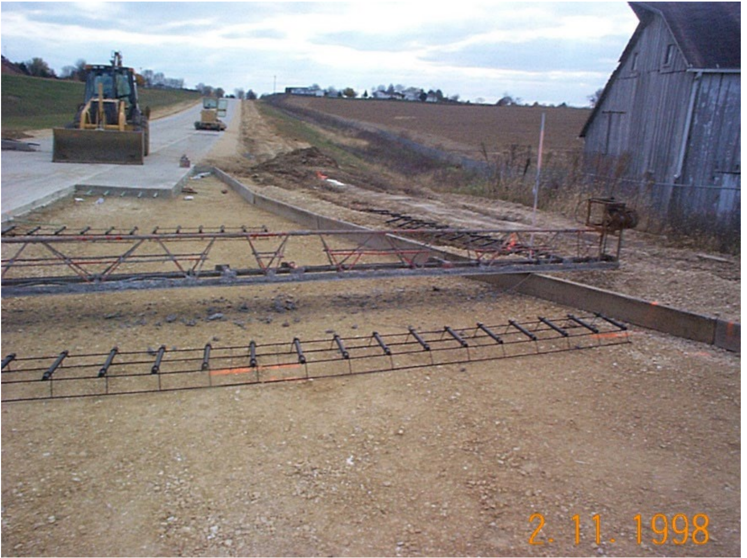
Fixed Form Paving
