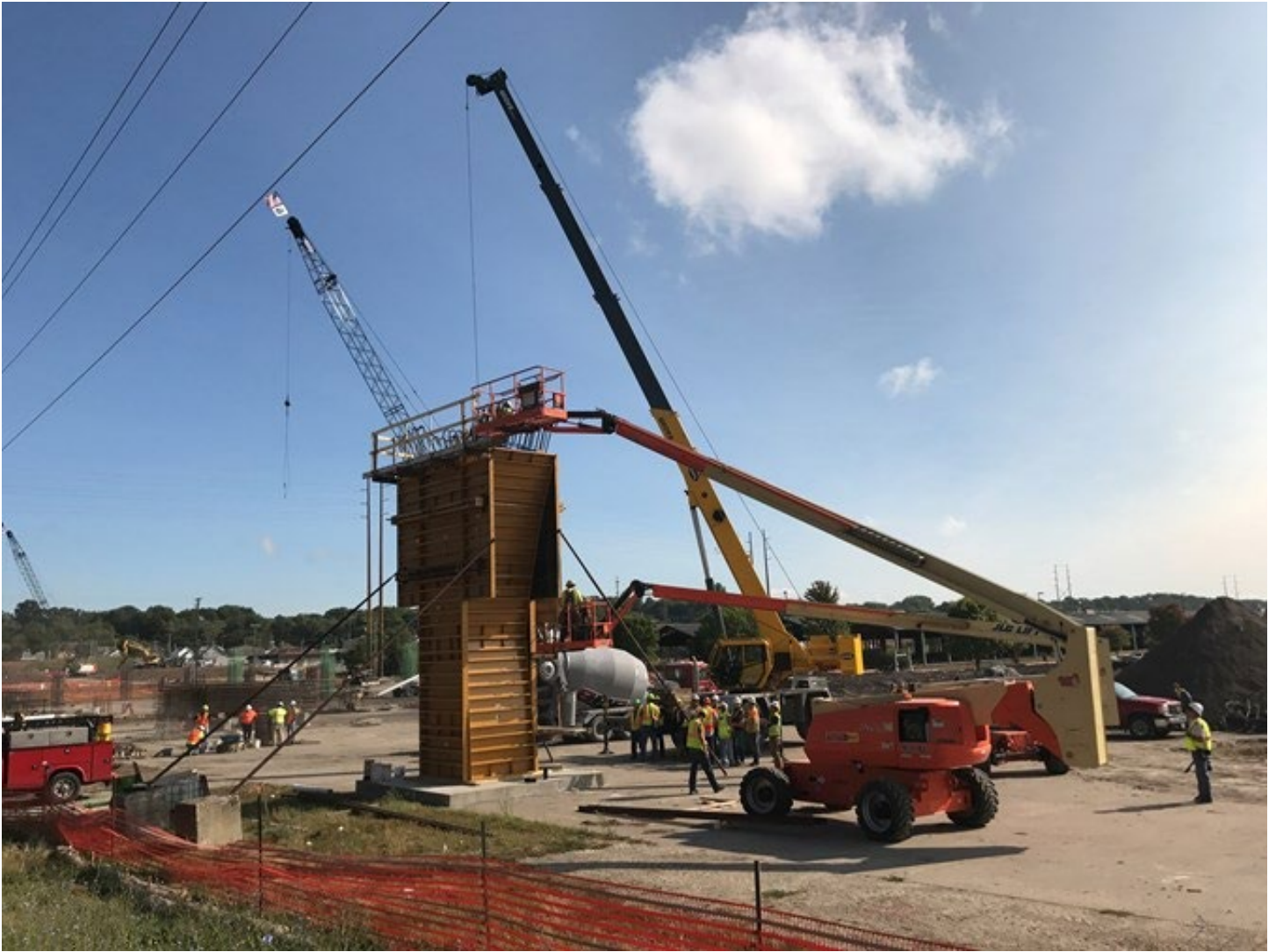
Pier Concrete Placement (Sub Structure)
