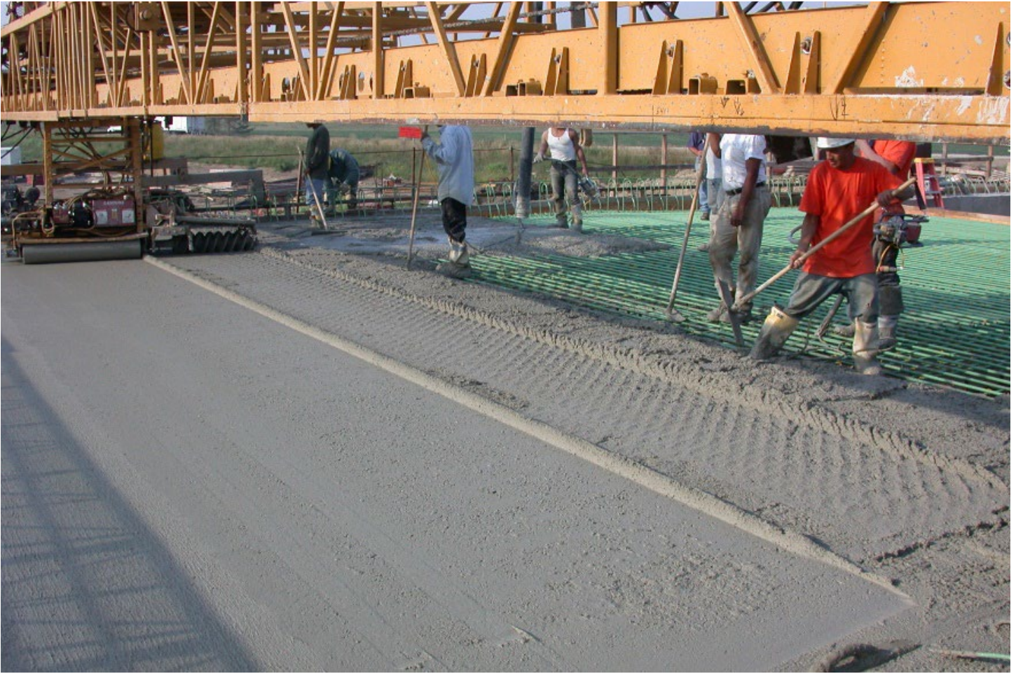
Bridge Deck Placement (Superstructure)
