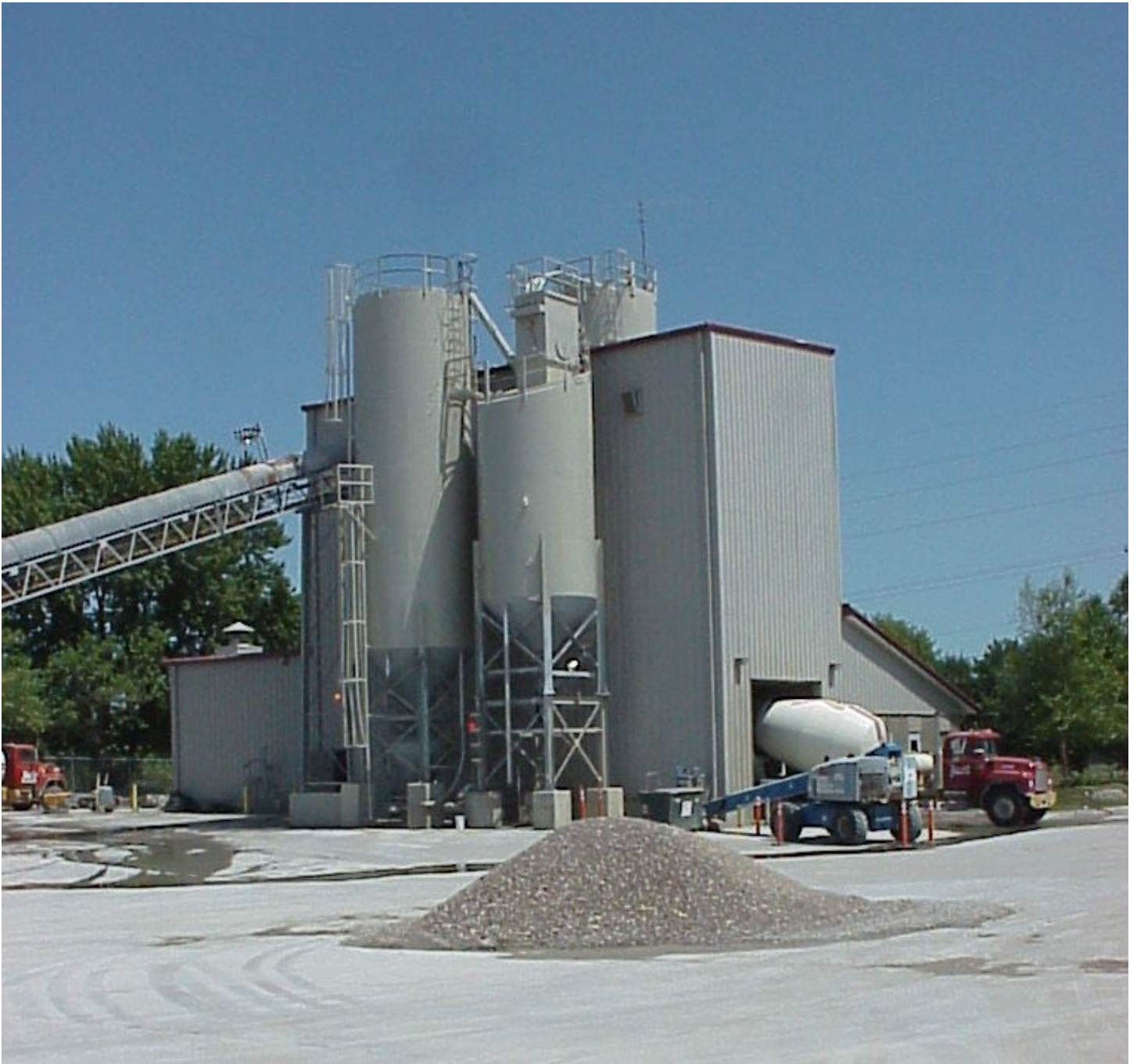
Ready Mix Dry Batch
