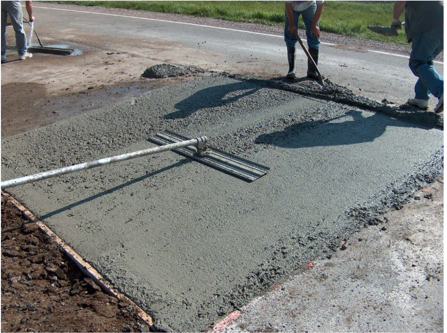
Full Depth Patching
