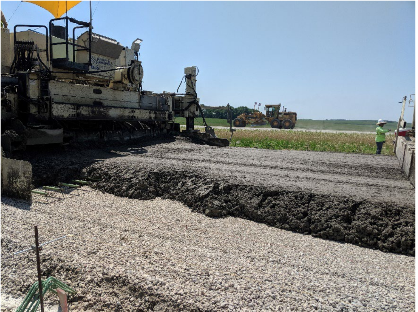
Slipform Paving
