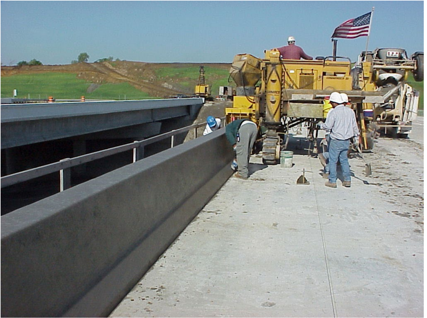
Slipform Barrier Rail
