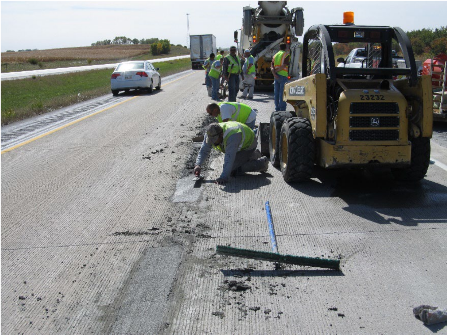
Partial Depth Patching
