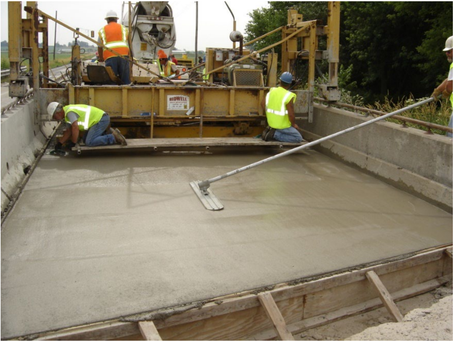
Bridge Deck Overlay
