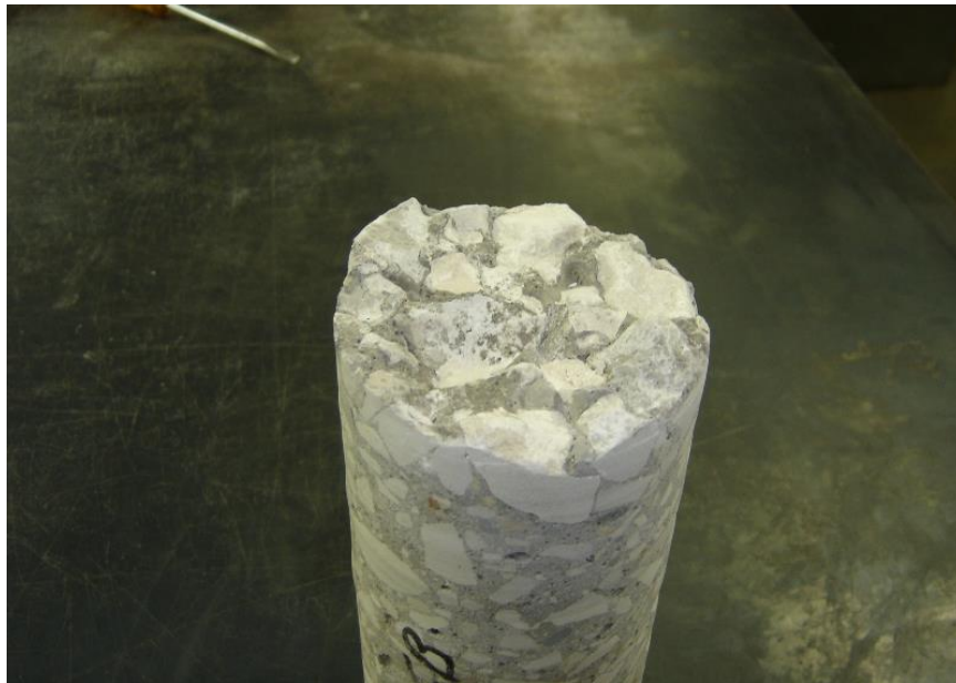
Figure 3. Concrete core with granular subbase removed.
