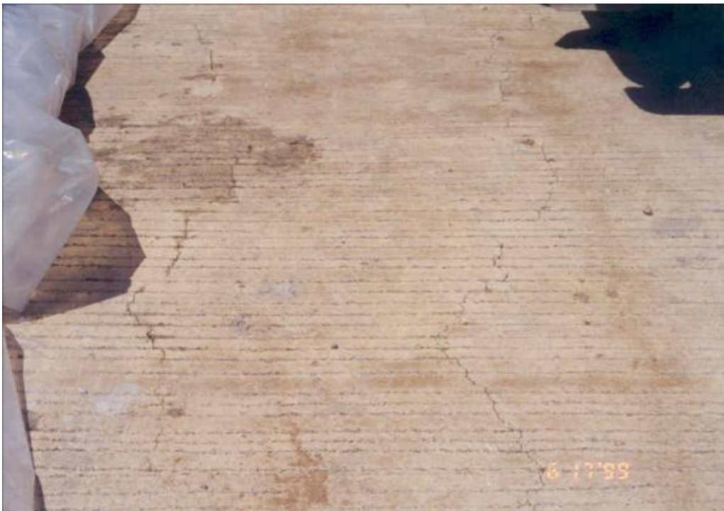
Figure 2-26 Plastic shrinkage cracks form perpendicular to wind direction
