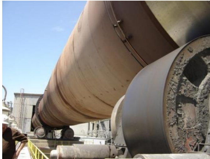
Figure 2-7 Kiln for cement production
