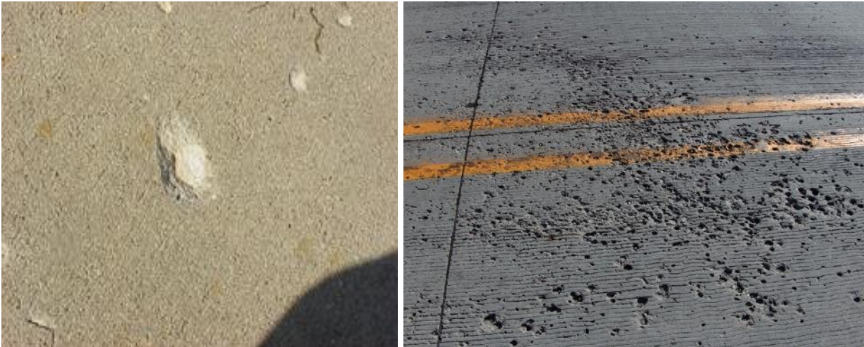
Figure 4-8 Oolite pop outs(left) and shale/chert pop outs (right)
