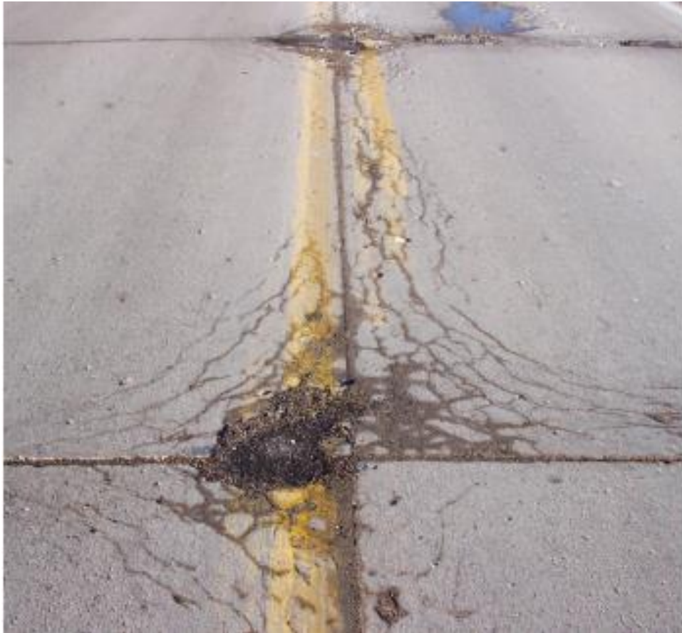
Figure 4-7 D-cracking deterioration
